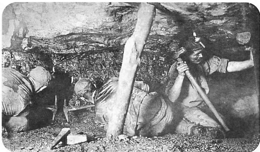
Victorian miners in the Rhondda (S. Wales) used naked flames which caused explosions due to 'firedamp' (inflammable gases) Source: bbc.co.uk
