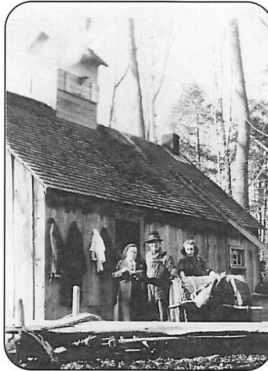
The house at Douglas Corners at the time of Céphas Péron. Source: author
