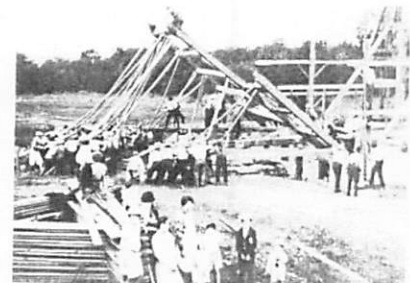
Erecting a bent of J B White's barn — Courtesy Ed. White
