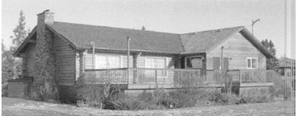
The Memorial Building, current home of the Southern Alberta Pioneers and Their Descendants - photo Gordon Lane
